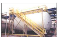
electrical utilities but have increasingly gained acceptance for general industry & residential uses. Composite ladders are stronger than wood or aluminium and do not absorb water, rot or corrode. The products could be pigmented with a suitable colour along with the resin during the pultrusion process. With the colour throughout the part, there is no chipping or peeling.
