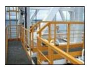
Source: Transocean Sedco ForexHandrails, ladders and gratings made with pultruded or molded composite materials require less maintenance and mean significantly less topside weight.
